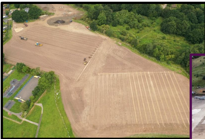
Progress at Grasmere Sports pitches
