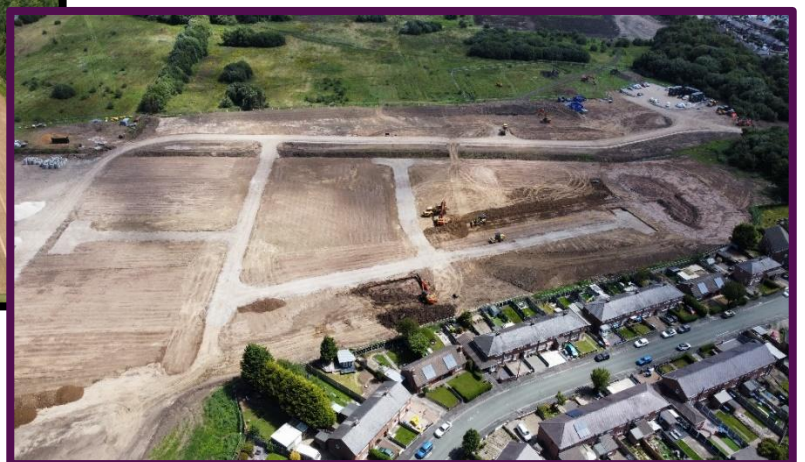
Groundwork at Poplars Avenue
